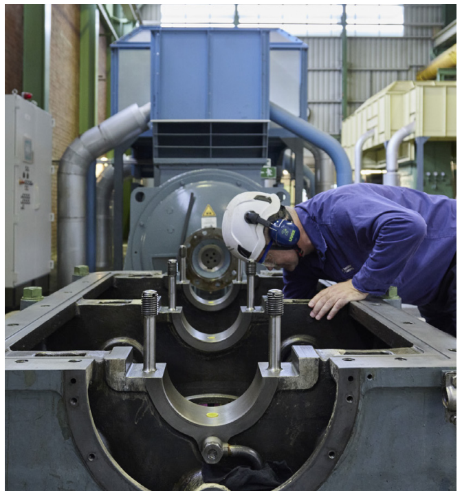
Structured solutions, including sealing material upgrades, can be delivered on site
