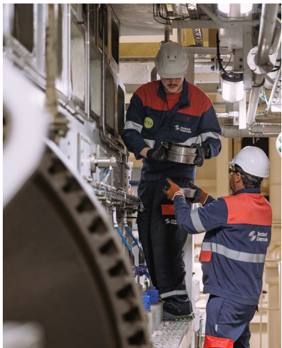
Compressor maintenance during dry-dock.
