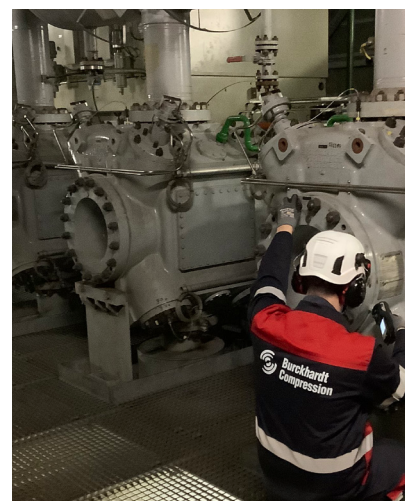
Local Burckhardt Compression field service representative during a detailed on-site inspection.
