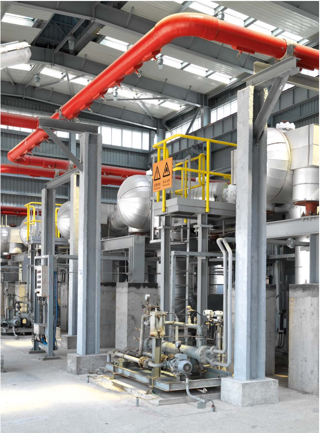
Three Laby® Compressor systems for BOG application at a Chinese LNG terminal
