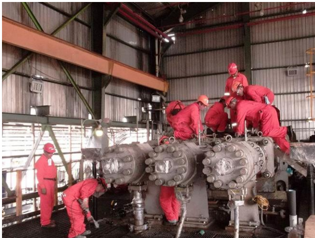
Disassembly of F6 Compressor by Burckhardt Compression
