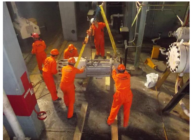
Dismantling of Cylinder, 2nd Stage by Burckhardt Compression
