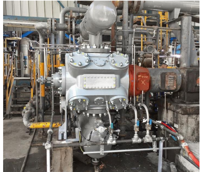
New cylinder of Burckhardt Compression designed according to API 618 5 th edition during the revamp service installation.
