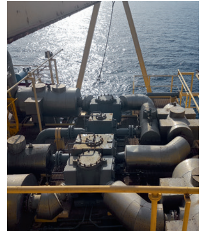
Laby®-GI Compressor as minimum-send-out on the FSRU vessel
