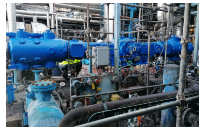
Repaired compressor being installed on site
