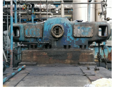
Old compressor frame on site before repair
