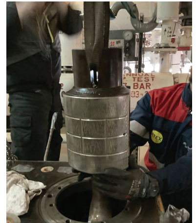
Installation of 2 nd -hand cylinder
