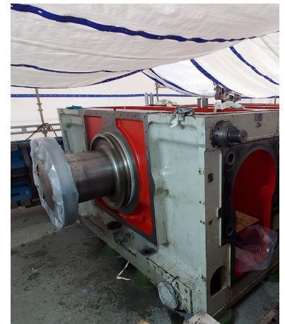
Installation, leveling & measurement of both crankcases were done in separate tent on site to keep temperature level stable.
