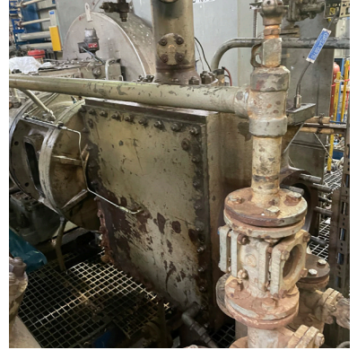
Compressor cylinder before replacement
