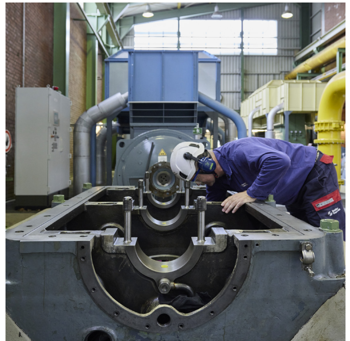
Image 3: Structured solutions, including sealing material upgrades, can be delivered on site.
