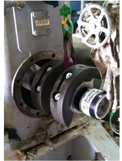
Installation of new crankshaft
